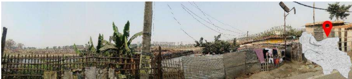
Figure 15 Unauthorised construction on the river floodplain
