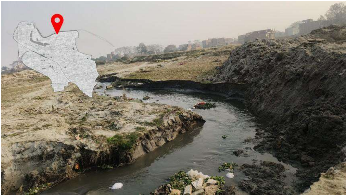
Figure 19 Major Outfall of the Chandwara Nallah near Siddhi Ghat
