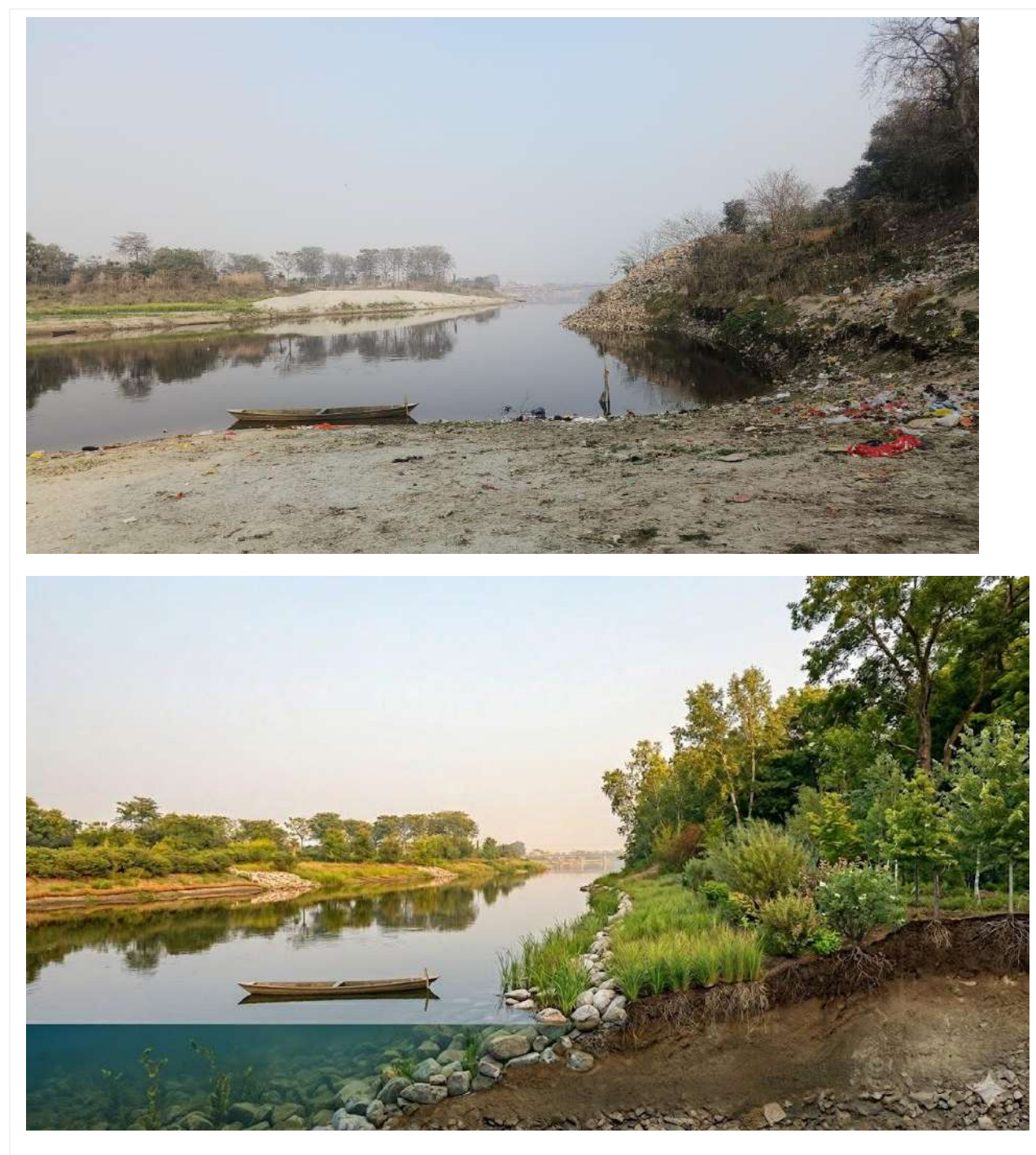
Figure 49 Before and After images of Edge Treatment and Stabilization
